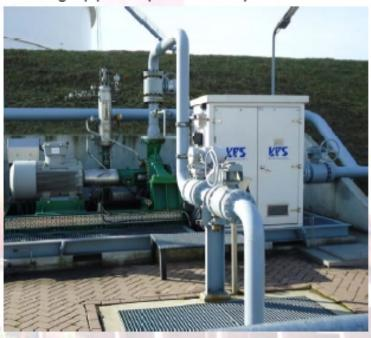
To achieve this a suitable pipeline location must be found or created at which the fluid is thoroughly mixed. Relying on natural turbulence for mixing is frequently not possible as this depends on maintaining minimum flow-rates. Rapid mixing may be essential, therefore a mixing system is required which provides adequate mixing regardless of flow conditions.
