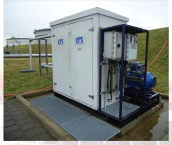
reducing the amount of hot tapping required on the main line. A KPS byscoop is placed in the central third of the pipeline, allowing for a representative flow to be transported to the KPS flowthrough CS-01 cell sampler.
